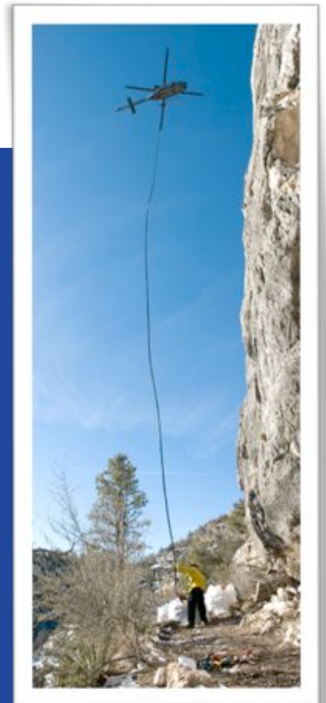
Helicopter at work on the Island Trail.
